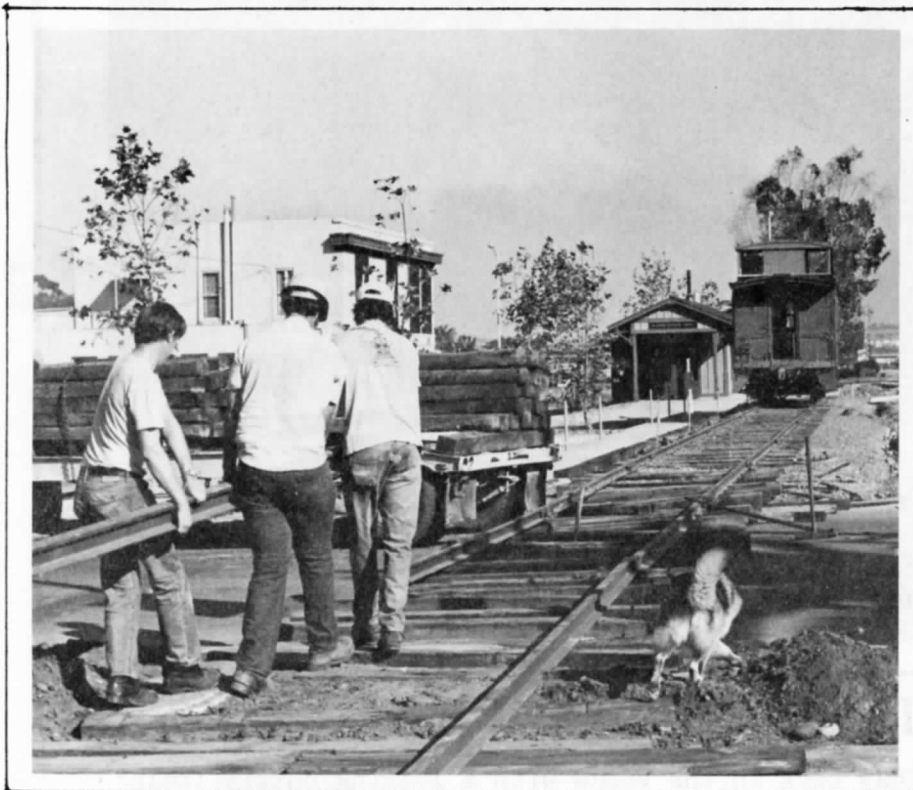
Museum regulars Bill Barbour, Dan Robirds, and Jim Lundquist, (left to right) are shown here placing the last rail for the temporary track across Lemon Avenue. The fuzzy tail at the right belongs to Jim's mutt "Ms. Sport", who has been a regular supervisor at PSRMA work sessions for the last few years. ATSF caboose #1413 and the south end of the La Mesa Depot are in the background.
