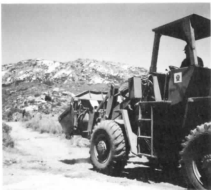
Allan Andrews clearing access road.
